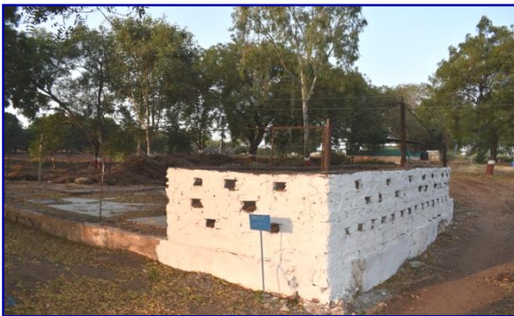
Nadep Compost Unit
