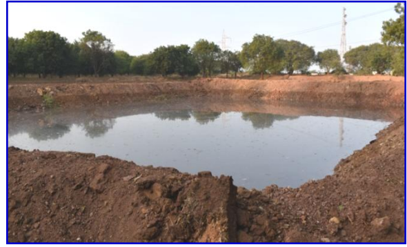
Water Storage Pond
